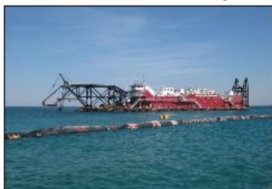
Dredge Texas at Boca Raton
