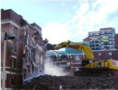
Demolition of Massachusetts Mental Health Hospital
