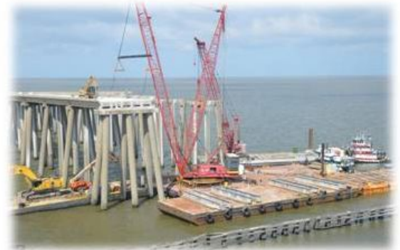
I-10 Bridge Project in Louisiana
