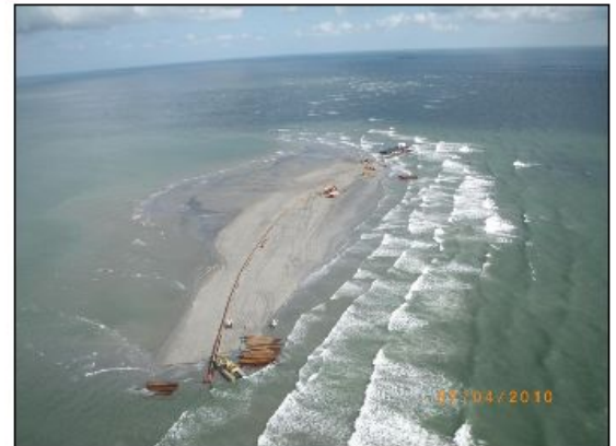
Berm construction off Louisiana coast
