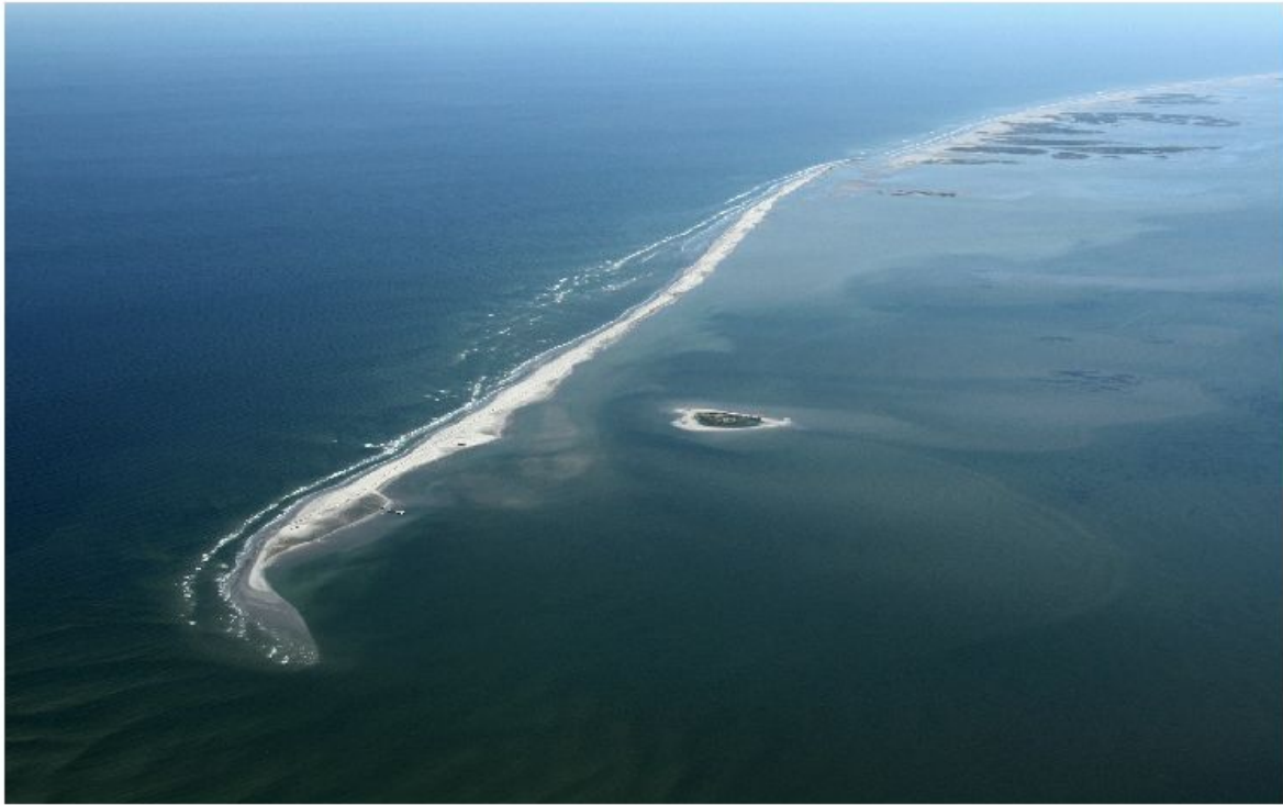
Berm construction off Louisiana coast
