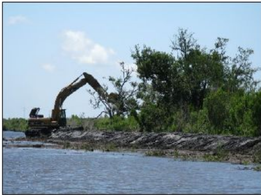
Bayou Dupont, LA Coastal Restoration
