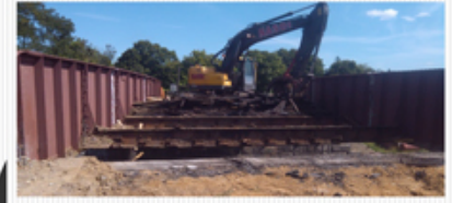
EXPANDING DEMOLITION BUSINESS
