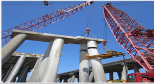
I-10 Bridge Project in Louisiana
