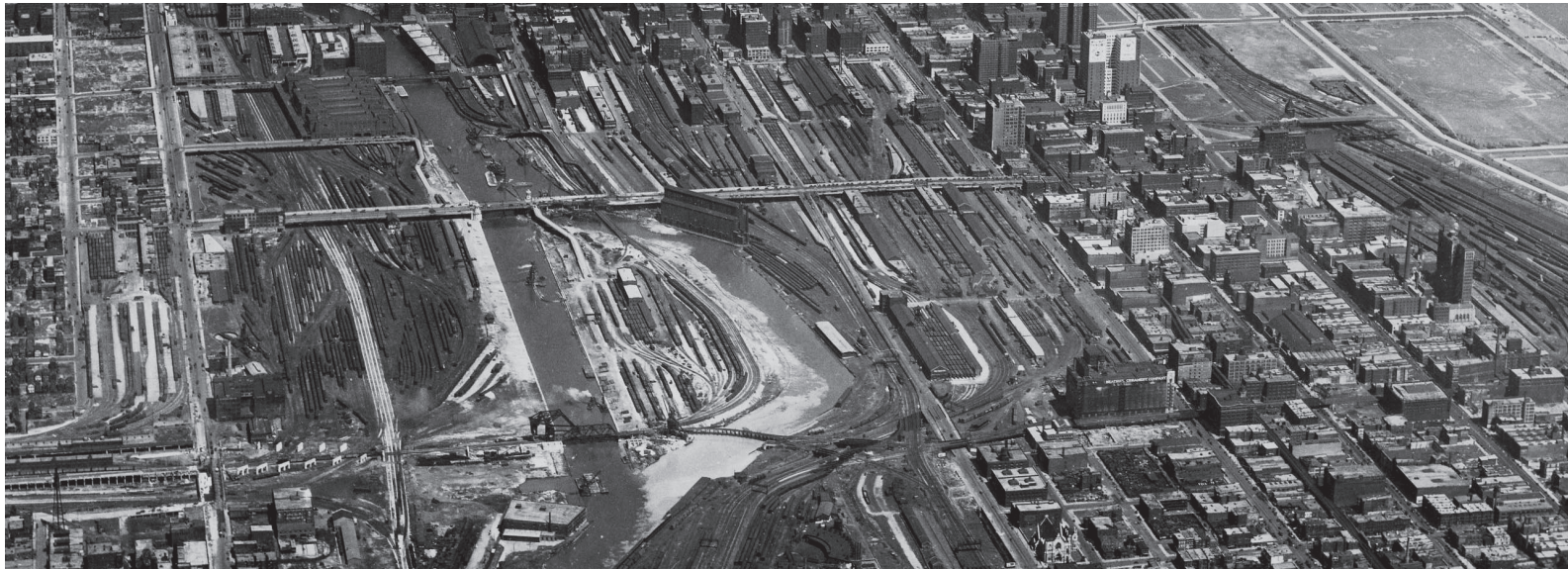
Straightening the south branch of the Chicago River, shifting the channel a quarter-mile west, 1930.
