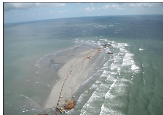
Berm construction off Louisiana coast
